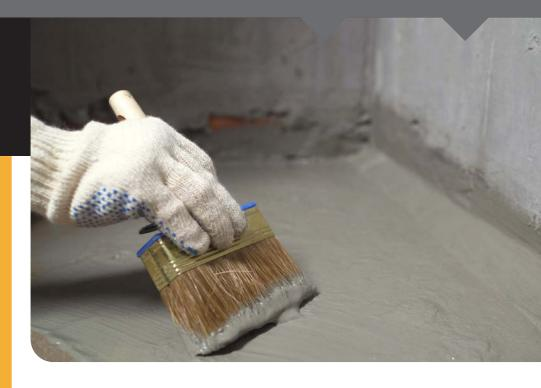
SBR Latex is a styrene butadiene copolymer latex, specially modified to be compatible with cement based mixes including ordinary portland cement or high aluminium cement. It may be incorporated into cementitious renders, screeds or patching mixes
