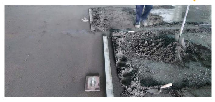
20 mm aggregate - 2.5 parts - 125 Kg by volume SBR Latex and water at 1:3 (or as required) Approximate mix volume = 0.14 m³ per 50 Kg of cement.
