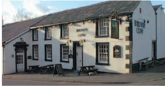
Work carried out by Turner Presentations.
