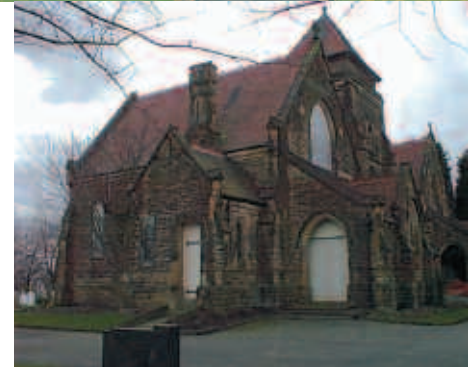
Urmston Chapel, Manchester. Work carried out by Protim.
