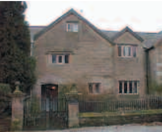
Work carried out by UK Remedial.
