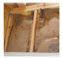
Compressing fiberglass diminishes its insulating value. When hard-to-fill gaps are stuffed with fiberglass, the result is a poor air seal. FROTH-PAK<sup>™</sup> products uniformly fill in gaps and maintain their original shape.
