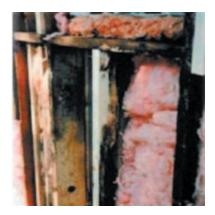
When wet, fiberglass loses insulating value, and it can provide suitable conditions for mold and mildew growth. FROTH-PAK<sup>™</sup> foam resists moisture, reducing the potential for mold and mildew growth.
