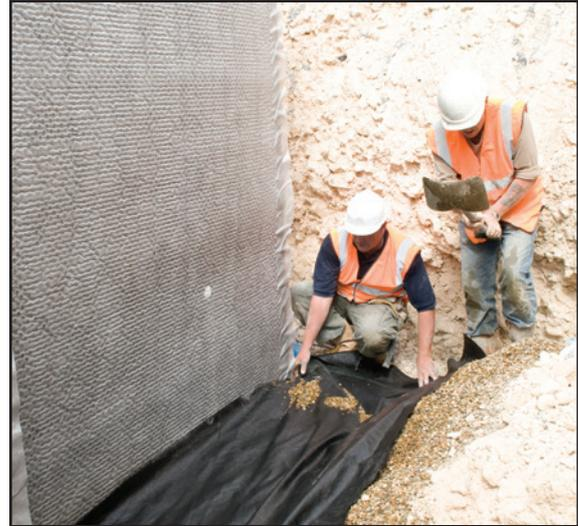
**Note:** Geotex drainage performance is dependent on water table levels. If the resting water table level rises above the drain level the cavity between the membrane and the wall will hold water and for this reason we recommend the primary paint-on waterproof coating is always applied to the foundation.
