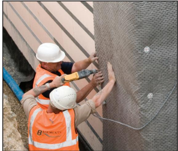
Fig 4: Fixing Membrane around corner
