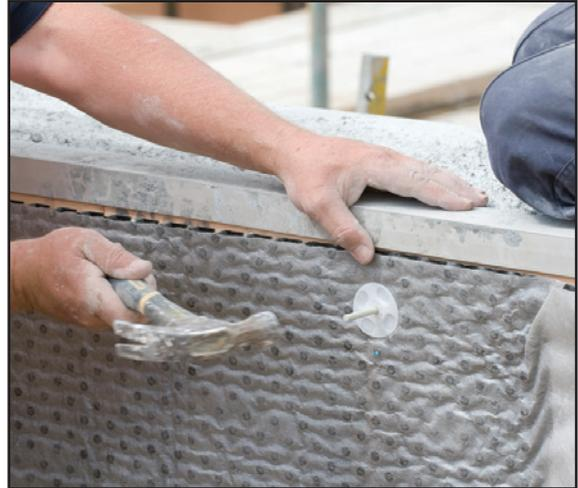
Fig 2: Fix Membrane
