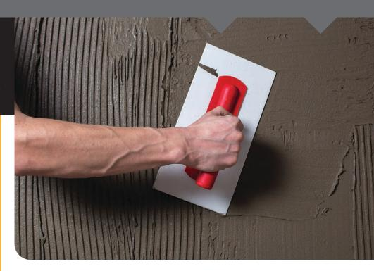
Wykamol **Renovation Plaster** is designed to have similar properties to a 1:1:6 cement:lime:sand plastering mortar. Lightweight, perlite aggregates replace a portion of the sand to reduce heat loss and condensation.
