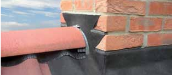
Photograph taken at BRE immediately after 49m/s (110mph) wind tunnel test
