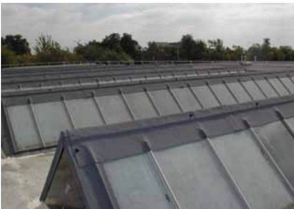
Flashing to a Northlight
