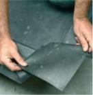
Adhere the membrane with bonding adhesive to the upstand and on top of the roof edge.
