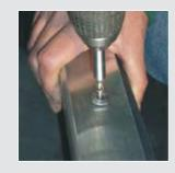
Attach the roof trim using stainless steel screws and neoprene rings.
