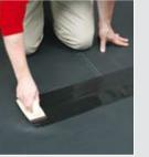
Apply QuickPrime Plus to both sides of the joint to a total width of 20 cm and wait until it is dry to the touch.
