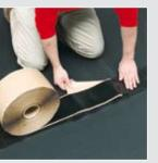
Pull the release paper at a 45° angle from under the QuickSeam Cover Strip and adhere the strip with a flat hand to the membrane. Make sure no air bubbles are trapped inside.
