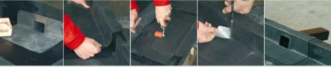
Place the RDP, press firmly in the Adhere QuickSeam SA Flashing Roll on with a hand roller. slope angle and screw it tight to over the RDP and onto the the substrate. Apply OuickPrime membrane. The strip should Plus to the top of the RDP and at overlap the edges of the RDP by at least 10 cm around the RDP. Allow least 5 cm in all directions. to drv.
