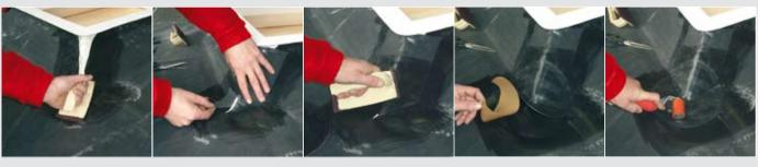
Cut the membrane from top to Adhere a piece of QuickSeam Apply a new layer of QuickPrime bottom up to the base at the external SA Flashing up to the base. Plus. corner. Adhere the membrane with Bonding Adhesive to the upstand. Apply QuickPrime Plus across 10 cm on both sides and allow to dry.
