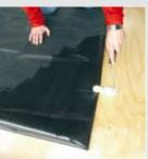
Apply Bonding Adhesive to the underside of the folded membrane
