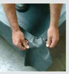
Fold the membrane flat onto the roof edge. The edge is finished with roof trim (see edge finishing) Excess membrane is trimmed off.
