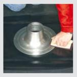
Apply QuickPrime Plus to the membrane (min. 10 cm around vent) and to the flange of the vent. Allow to dry.
