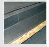
Adhere the QuickSeam SA Flashing to the gutter, Roll on with a hand roller.
