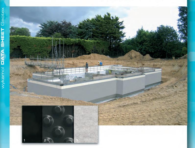
Wykamol Geotex is a multi-layered cavity drain membrane designed to prevent ground water penetration in any situation where internal walls are below external ground level (up to 10 m depth). It is designed for use on the outside of the building on vertical elements prior to back-filling.
