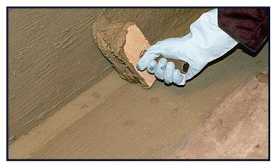
Cracks and bolt holes must be cut out and filled solid with NO MORE DAMP water stop prior to the application of NO MORE DAMP tanking slurry. Substrates contaminated with high levels of soil or ground water sulphates may require attention.
